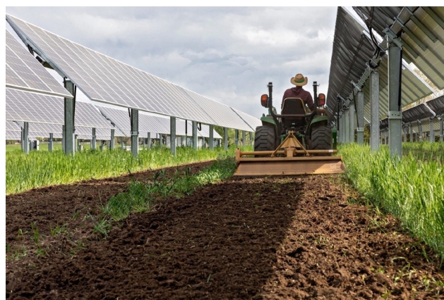
Fig. 2. The agrivoltaic system allows passage of the autonomous agricultural equipment (an example).
