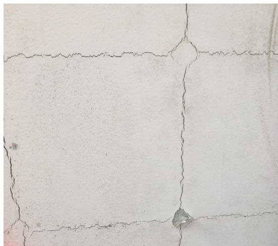
Fig. 1. PV panel back sheet degradation.
