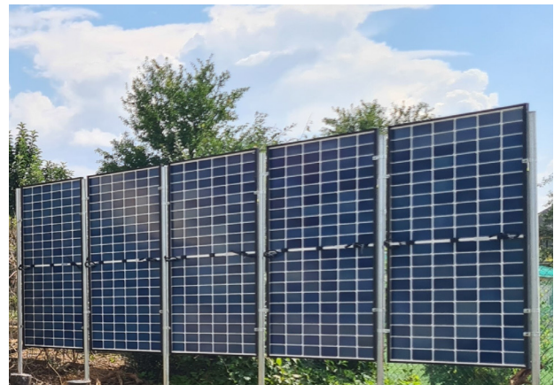
Fig. 5. Small agrivoltaic system with vertically arranged PV panels in the Czech Republic.
